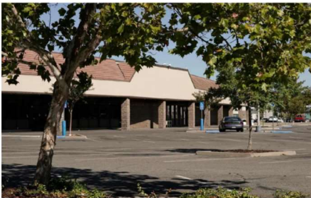
A commercial building sits empty in Sacramento, Calif., Thursday, Sept. 22, 2022. Two new laws in California will let developers bypass local governments to build housing on commercial land. Gov. Gavin Newsom on Wednesday, Sept. 28, 2022, signed a pair of laws aimed at increasing housing production in California. (AP Photo/Rich Pedroncelli)
