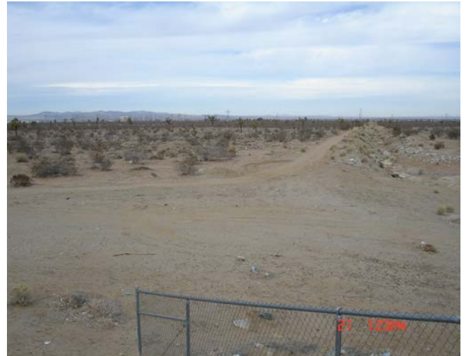
2. Looking northwesterly over the project site along the drainage channel from Mojave Drive bridge near center of site.
