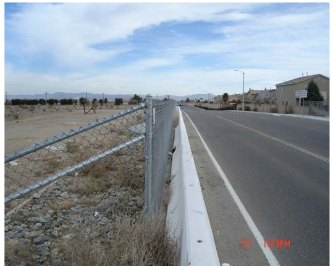
4. Looking east on Mojave Drive from the drainage course at the center of the project site.
