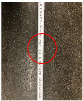
PEX Potable Water line with NSF- 61 label
