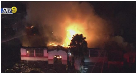
Fire crews battled a blaze at an abandoned school in San Bernardino Wednesday night. (CBSLA)
