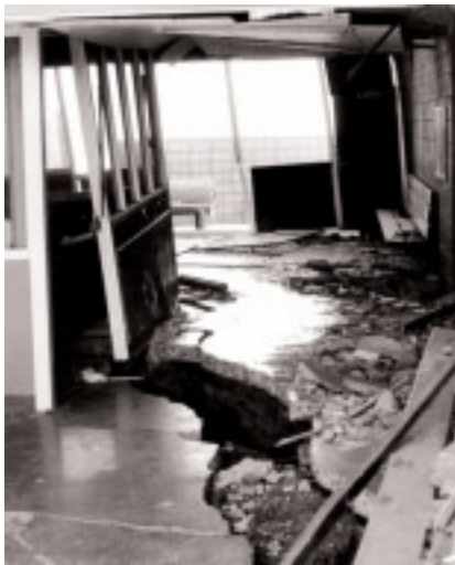
LA County Juvenile Hall, Sylmar, California damaged by liquefaction during the magnitude 6.6 San Fernando earthquake of February 9, 1971. Photo by Jack Meehan, structural engineer.
