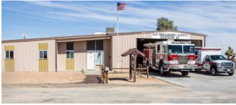
San Bernardino County Fire Station 42 in Downtown Yucca Valley
