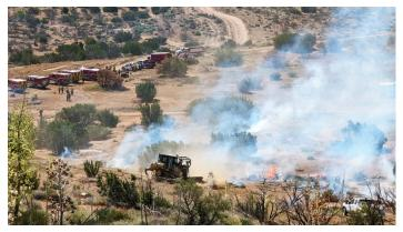
Bulldozers move dirt to create a fire line perimeter around the fire to prevent a forward spread.
