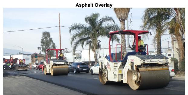
Finally, a structural section of one and one-half inches of rubberized asphalt concrete pavement will be spread and compacted to establish the new road surface. The new rubberized asphalt will reduce tire noise, smooth the surface, slow the appearance of future cracking, and improve the overall quality of the ride. After the new asphalt is placed, the pre-existing manholes will be raised to match the new surface.
