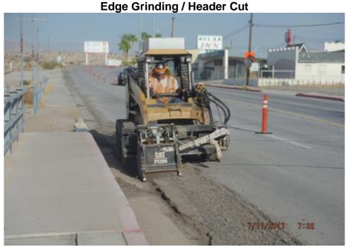
The first step is to reduce the existing height of the asphalt near the curbs and gutters, so that new materials will meet the surrounding materials at approximately the same height. At this same time any extremely rough or unstable areas of roadway will be addressed appropriately, and sidewalk ramps will be upgraded and constructed.
