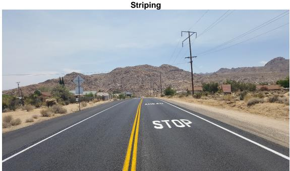
Approximately one week after the physical paving is completed, the final step of the construction will be to place new centerline, lane edge and stop limit line striping, along with new pavement markings.
