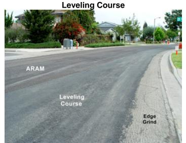
The next step will be to spread and compact a thin layer of asphalt on top of the existing road surface, filling cracks and fixing potholes. (ARAM - asphalt-rubber membrane interlayer shown in the picture above is the next layer).
