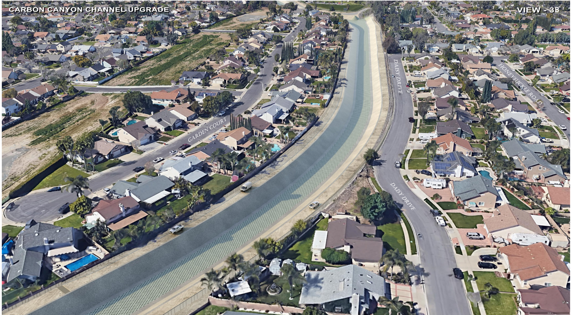
View before vegetation reestablishment in channel bed –new channel looking west along Daisy Dr.
