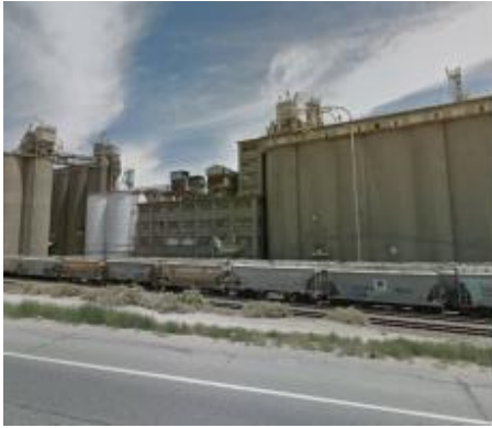
The CEMEX cement plant in Victorville, CA. Image courtesy of Google Maps
