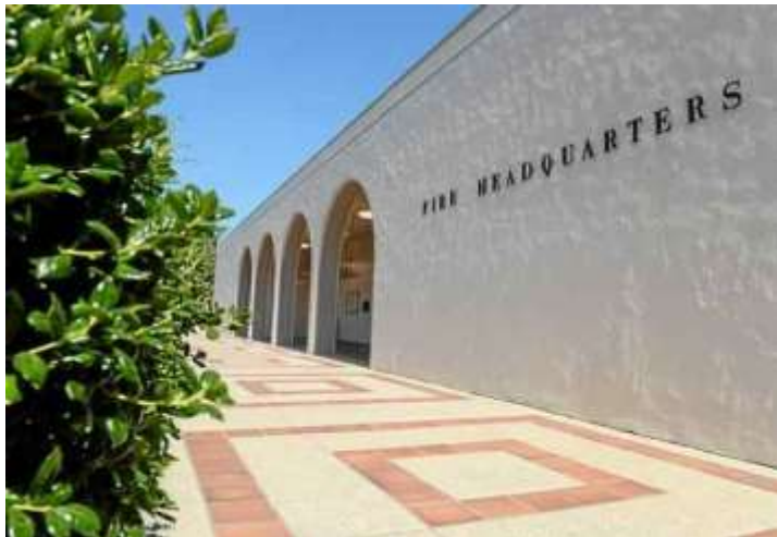
Upland Fire Station No. 1 is seen in a June 2013 file photo. (Jennifer Cappuccio Maher/Southern California News Group)
