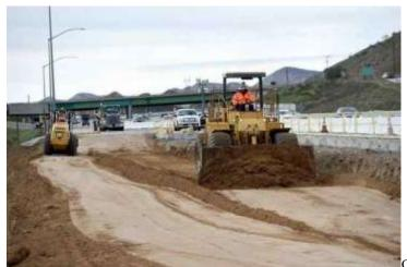
Construction crews work to repair four southbound lanes of Interstate 15 through the Cajon Pass, which sustained significant damage from last weeks heavy rain, Tuesday afternoon, February 21, 2017. A 200-foot section of the southbound freeway's No. 5 lane collapsed Friday night due to an overflowed creek weakening the road's base, according to a Caltrans news release. A big-rig and a San Bernardino County fire engine were taken out during the collapse.(Photo by John Valenzuela/The Sun)
