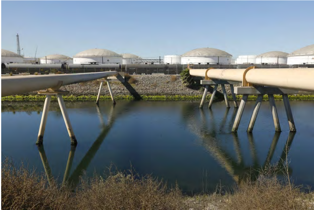
Fuel pipes cross the Dominguez Channel, where four months ago a warehouse fire sent millions of gallons of hand-sanitizer liquid laced with carcinogenic substances sloshing into the channel, creating a putrid scent of sewage. (Carolyn Cole / Los Angeles Times)
