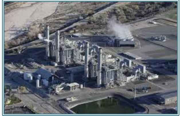
Southern California Edison's Mountainview Generating Station in San Bernardino County is one of the most efficient in the state . Although natural gas burns much cleaner than some fuels such as coal, this plant is one of the largest contributors of greenhouse gas emissions ( \text{CO}_2 ) in the state according to the Environment California Research & Policy Center.
