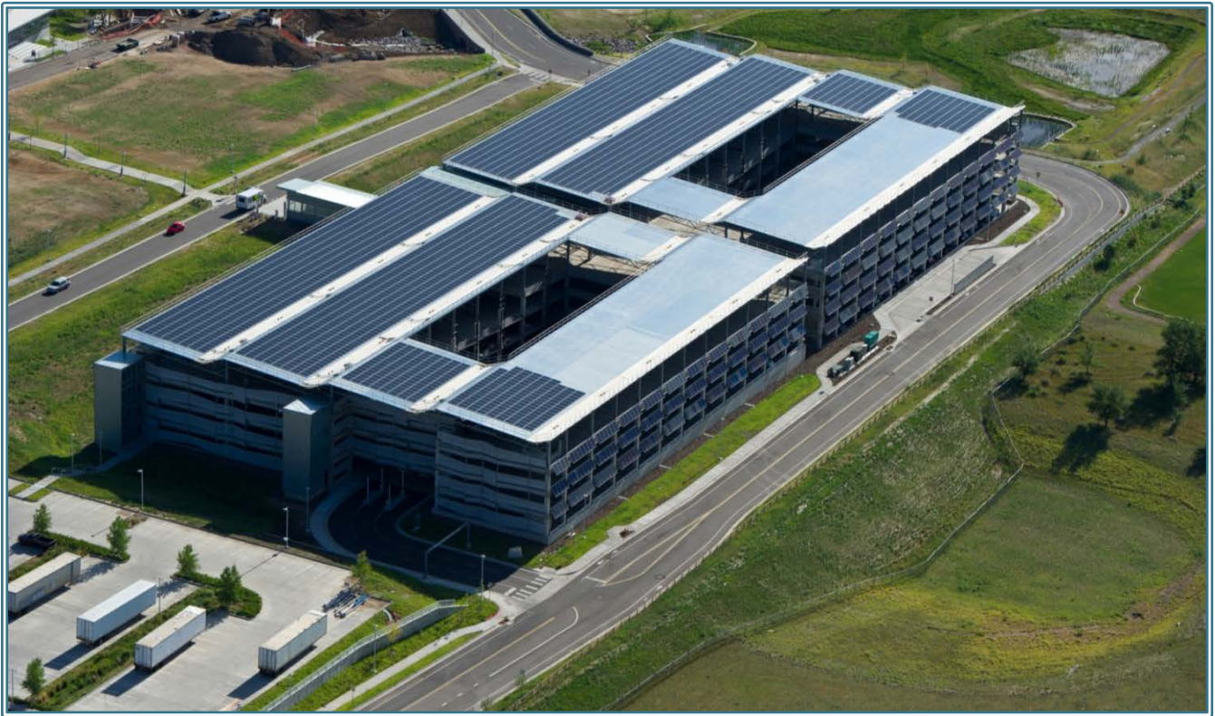
A parking garage at the National Renewable Energy Laboratory, with much of the roof space covered by solar panels. Government agencies can lead by example to demonstrate the feasibility of renewable energy installations, as well as energy efficiency and conservation practices (NREL 2012b).
