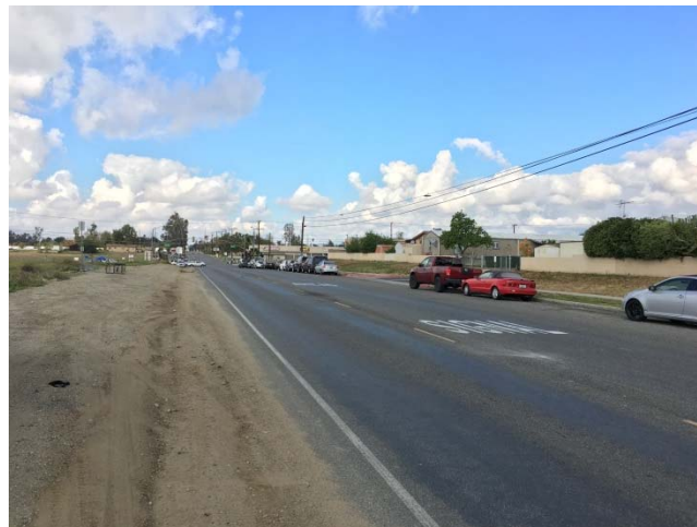
Northeast Corner looking west
