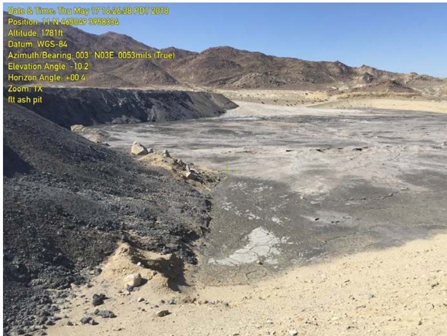
Exhibit 7: PVL Lime Plant location – Looking northeast from the center of the Southwest side of the project site - view of open Cell #5 showing disposed boiler ash
