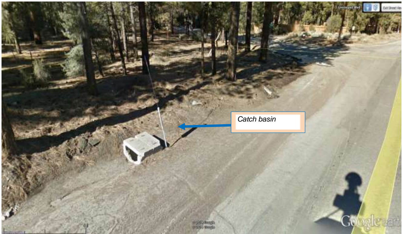
Catch basin just south of the intersection of Highway 38 and State Lane
