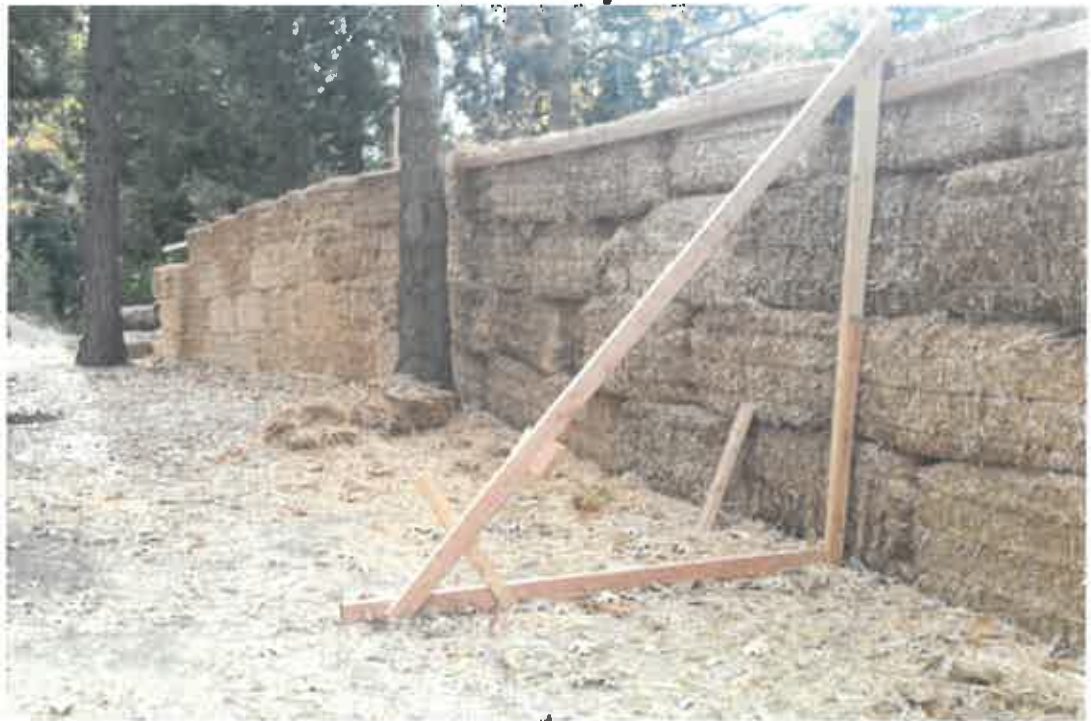
Figure 15 Sound Wall Hay Bales
