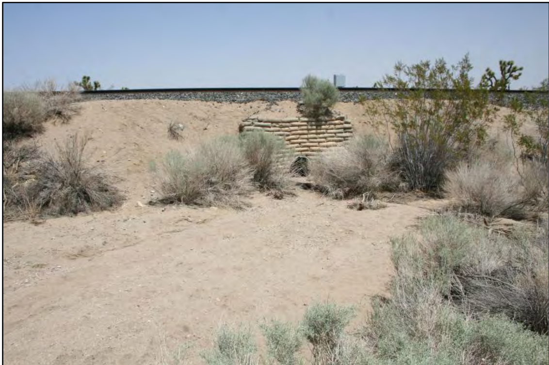
Photo 3 – View of downstream end of Drainage A where it exits the site through a 2-foot corrugated metal pipe beneath the railroad tracks at the north end of the study area.
