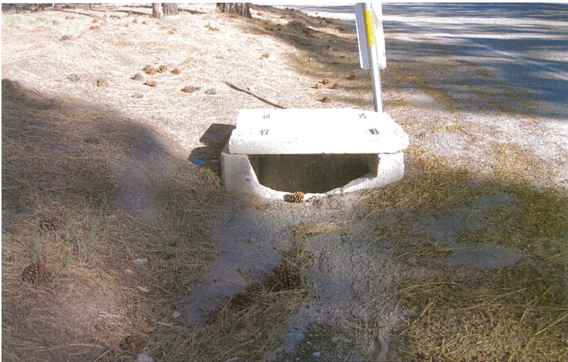
CATCH BASIN ALONG HIGHWAY 38 WEST OF SITE
