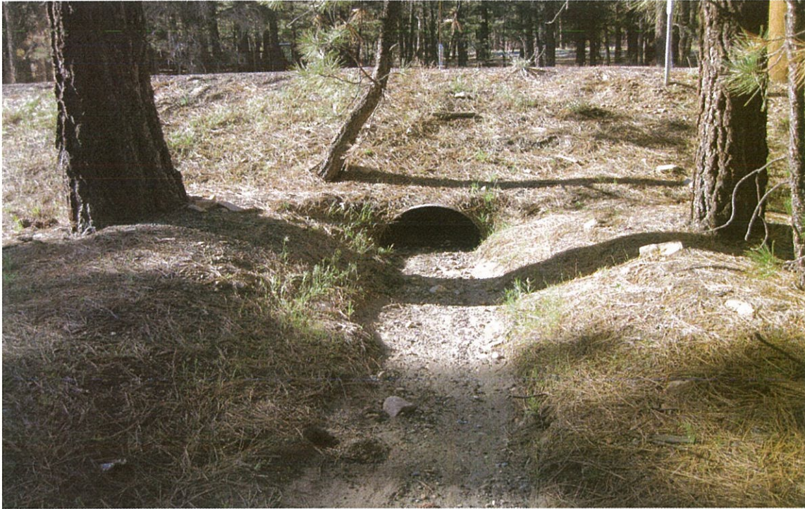
CULVERT UNDER HIGHWAY 38 LOOKING WEST
