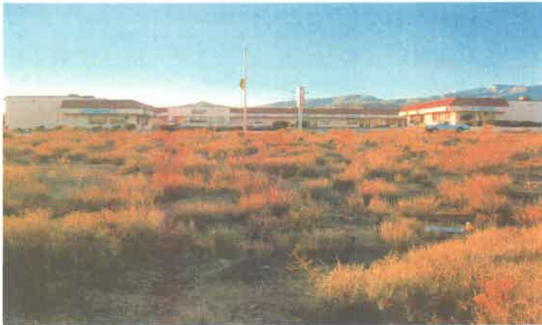
CENTER OF SITE LOOKING SOUTH
