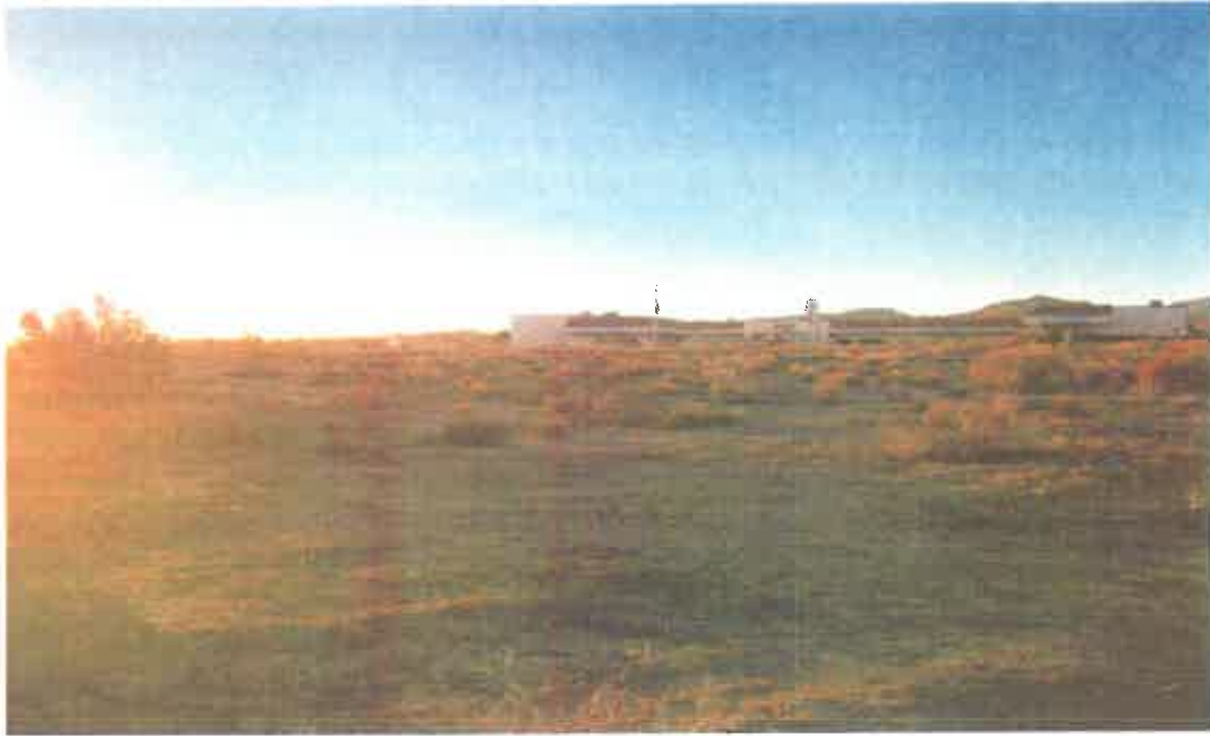
NORTHWEST CORNER LOOKING SOUTHEAST
