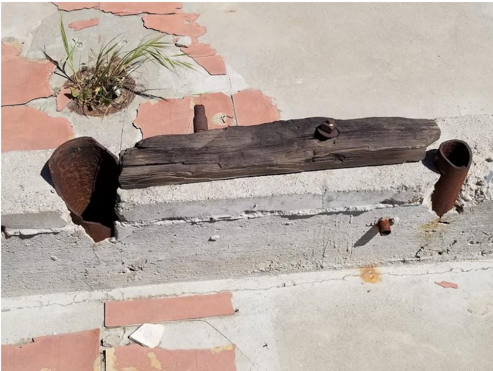
Photo 2: EMT1802-H-9, Feature 1 Footing Detail with Toilet Drain (View West)
