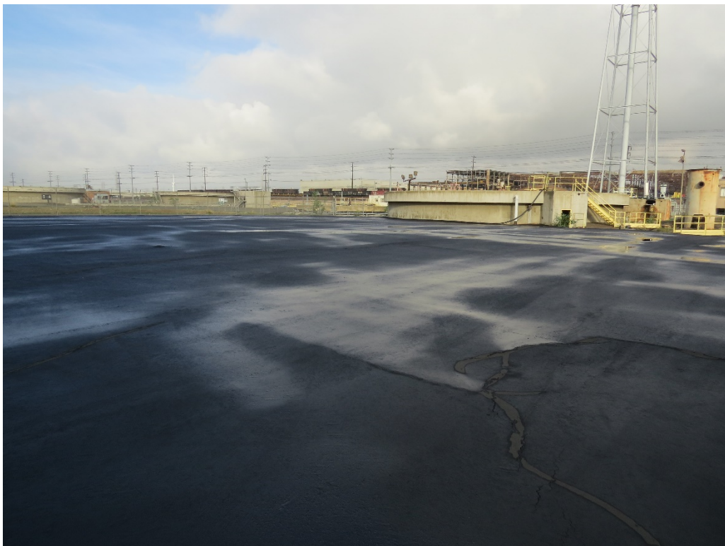
Photograph 8: From the southeast corner of the project site looking northwest.
