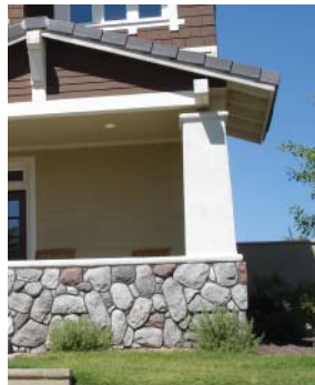
Walls of brick, siding, stucco, or stone
