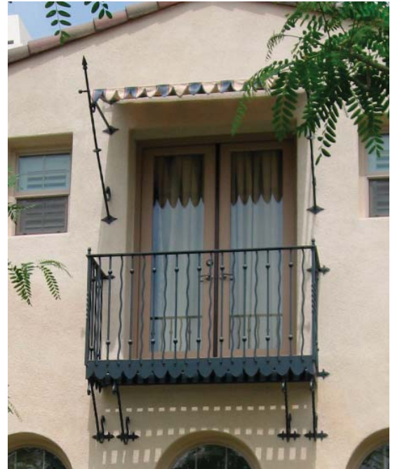
Wrought iron balconies
