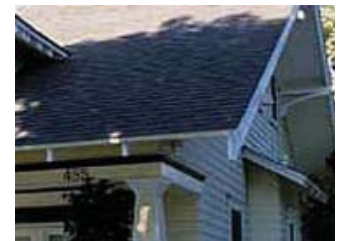
Flat tile roof
