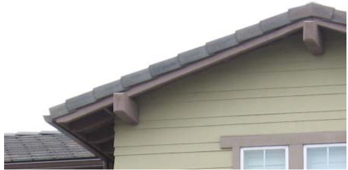
Exposed rafter tails
