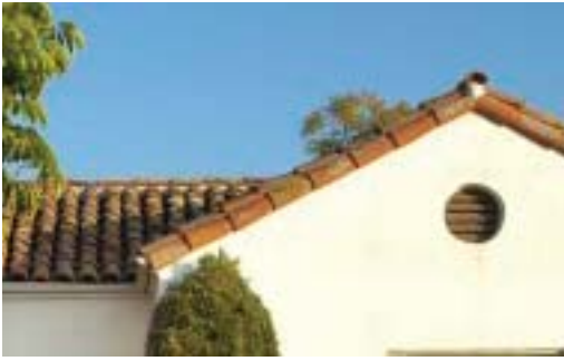
Red barrel tile roof
