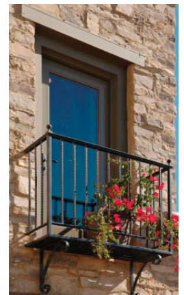
Wrought iron balconies
