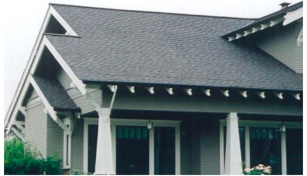
Exposed rafter tails
