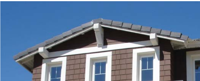
Decorative beams and braces below gables
