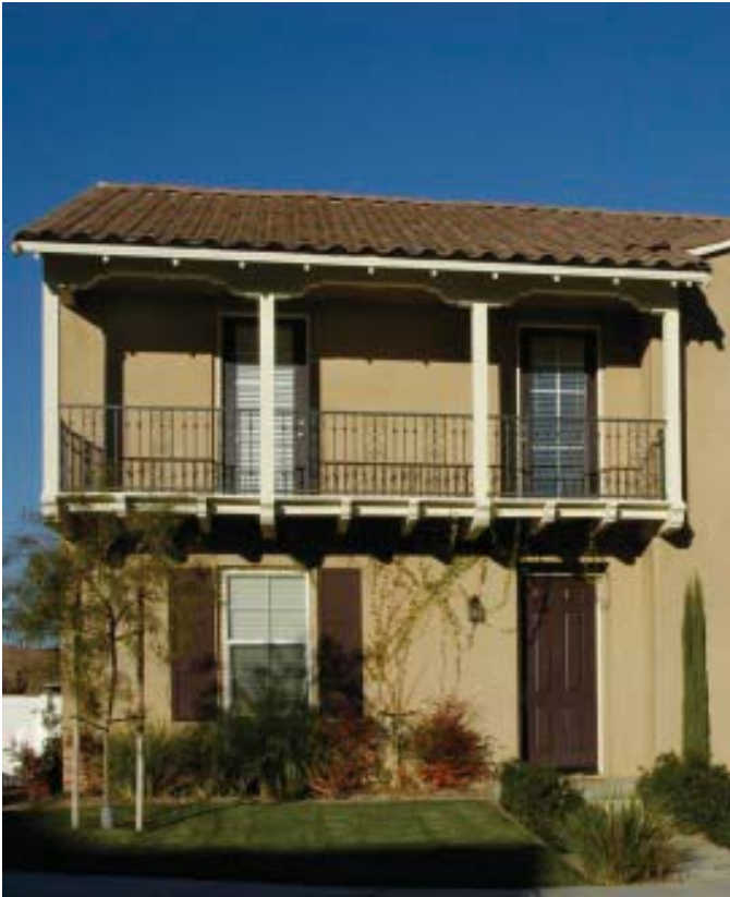
Cantilevered balconies along front facade
