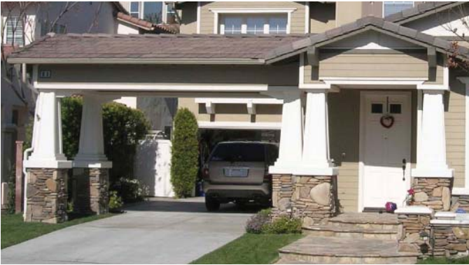
Horizontal emphasis of building forms
