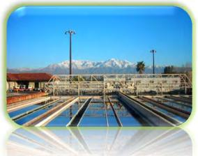
RP-2 is located in the southern service area in the City of Chino near El Prado and Pine Avenues and has been in operation since 1960. RP-2 wastewater flows have been diverted to Regional Water Recycling Plant No.5 (RP-5), and as a result RP-2 no longer processes wastewater. Instead, it treats the solids flow streams from the Carbon Canyon Water Recycling Facility, and Regional Water Recycling Plant No. 5 (RP-5) facilities.
