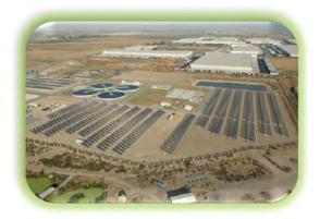
The installation at these sites includes different technologies: roof and ground mounted fixed-tilted panels, horizontal trackers, and tilted trackers. Tilted single-axis tilted tracker, installed at RP-5 just behind IEUA's headquarters, and pictured here, generate 30% more energy than fixed-tilt technology.
