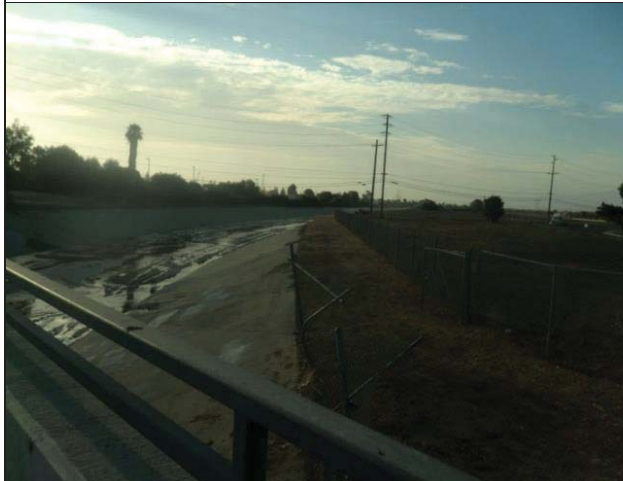
Photo 5: Concrete lined- flood control channel (Chino Creek).
