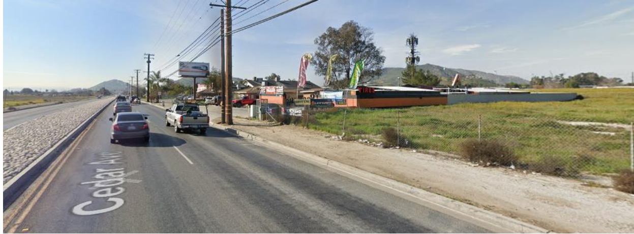
South View from Cedar Avenue
