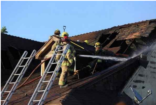
Firefighters mop up a house fire in the 1100 block of Bobbett Drive of San Bernardino Wednesday evening. Photo by John M. Blodgett
