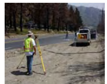
Surveying activity in Lytle
