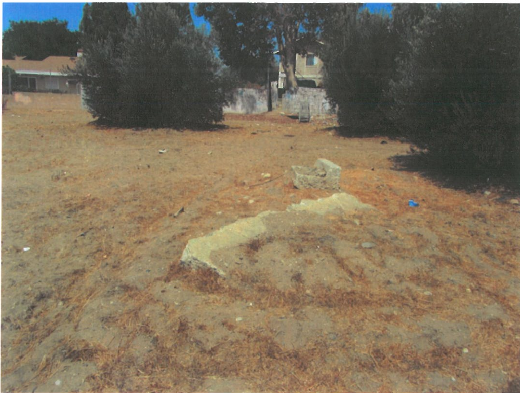
Photograph 6- Concrete rubble pile on the southern half of the project site.
