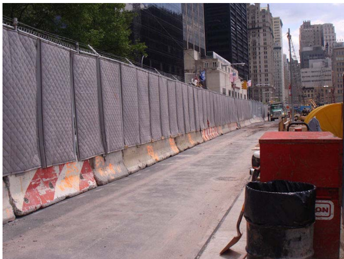
K-Rail Temporary Fence & Acoustic Material
