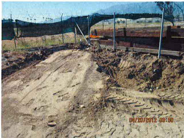
1. Western Excavation Area
