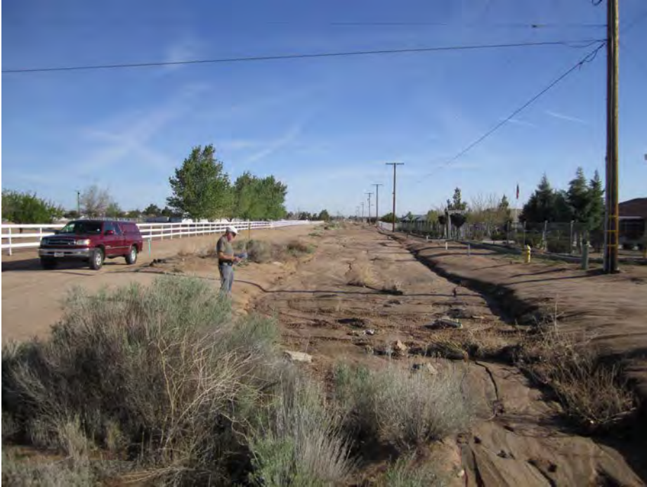
Looking northerly down Fuente Avenue. Standing near the northwest corner of the property. This erosion illustrates a fairly large volume has flowed in this location recently.
