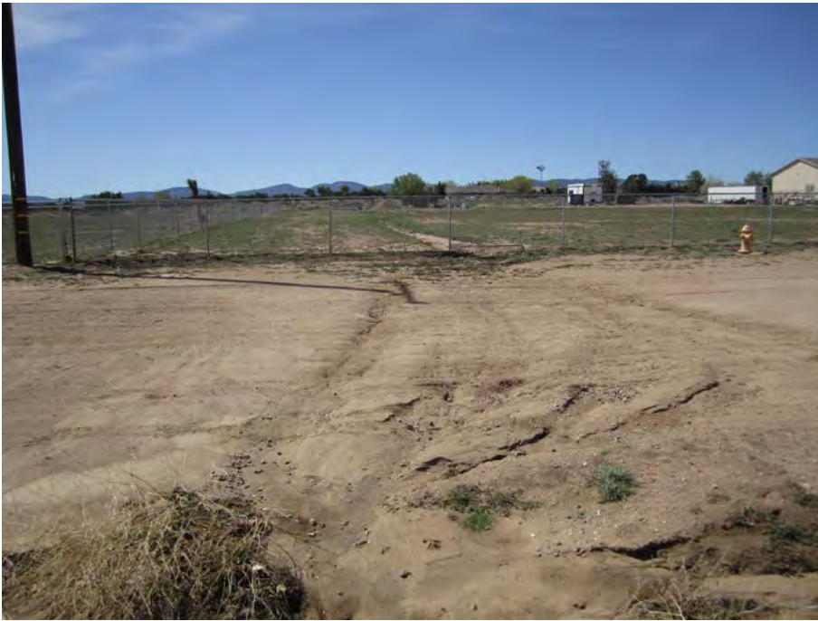
Looking southerly down the 84' drainage easement from approximately the midpoint of the southern property line on El Centro Road. This erosion illustrates a fairly low volume has flowed in this location recently.
