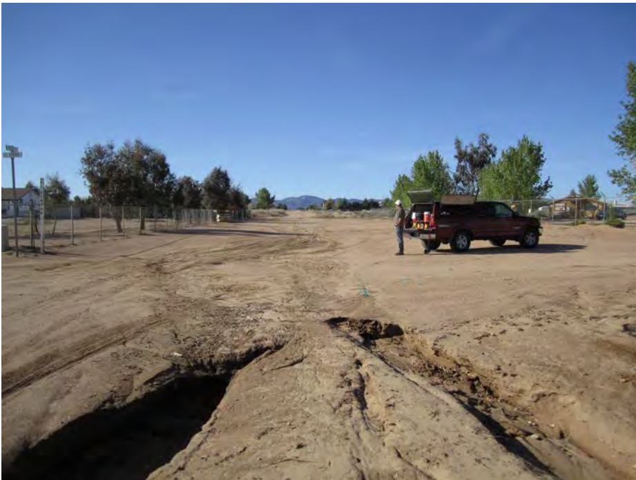
Looking southerly down Fuente Avenue. Standing near the southwest corner of the property. This erosion illustrates a fairly large volume is flowing from the south and the west at this location.
