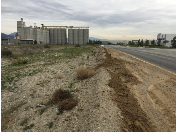
Looking east at southwest corner east of chain-link fence
