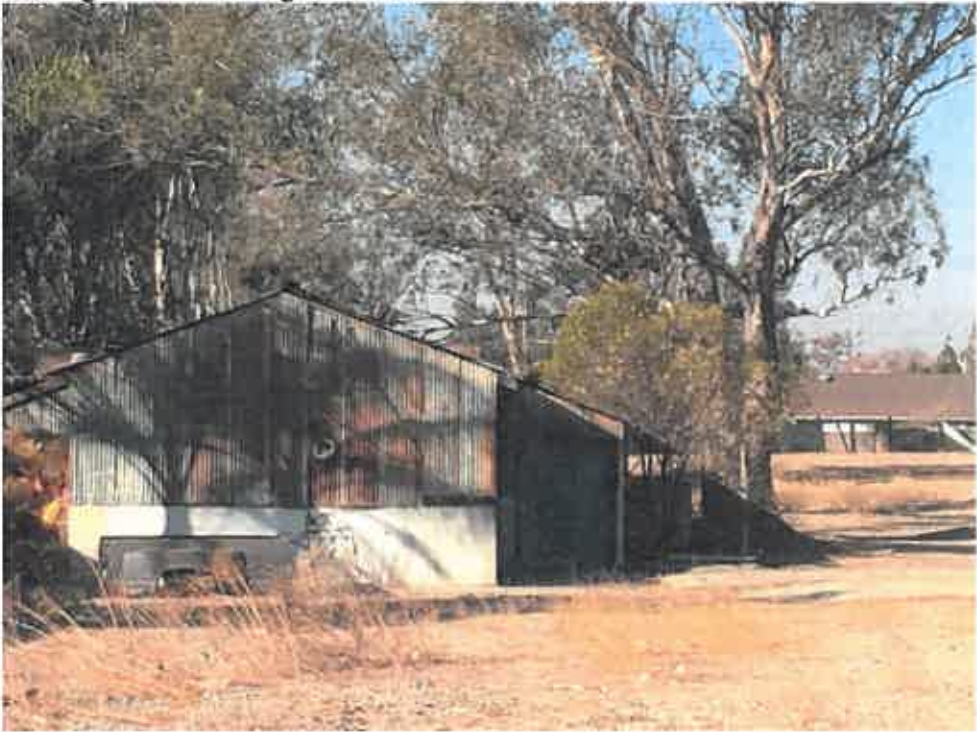
Photo 10: Existing structure along southern border in the middle of the site
