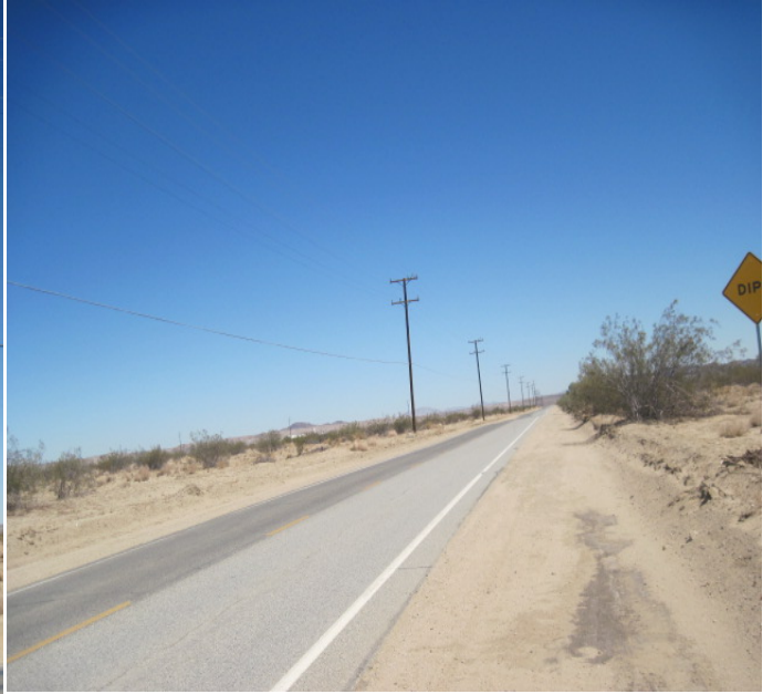
Photograph 10: Looking northwest at the generation line extension along Sunfair Road.
