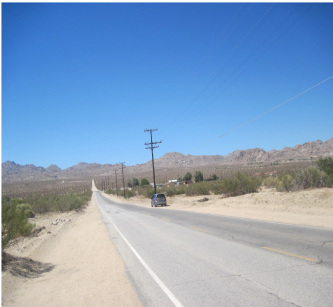
Photograph 11: Looking southwest at the generation line extension along Sunfair Road.
