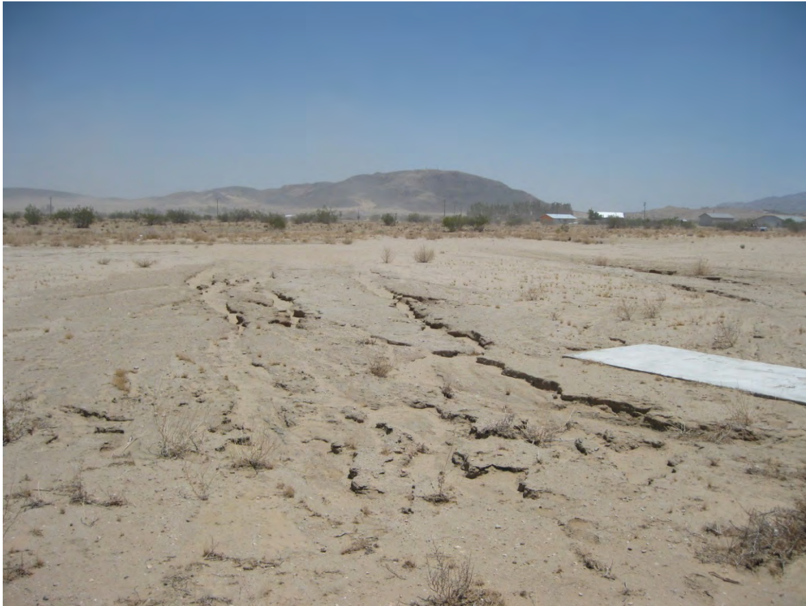
Photo 7: Erosion across graded dirt runway, looking northeast.
