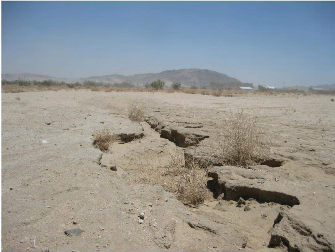
Photo 9: Erosion across graded dirt runway, looking northeast.
