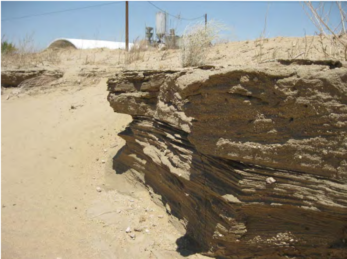
Photo 12: Offsite channel erosion downstream from berm pictured above. Vertical face approximately 18 to 24 inches high.
