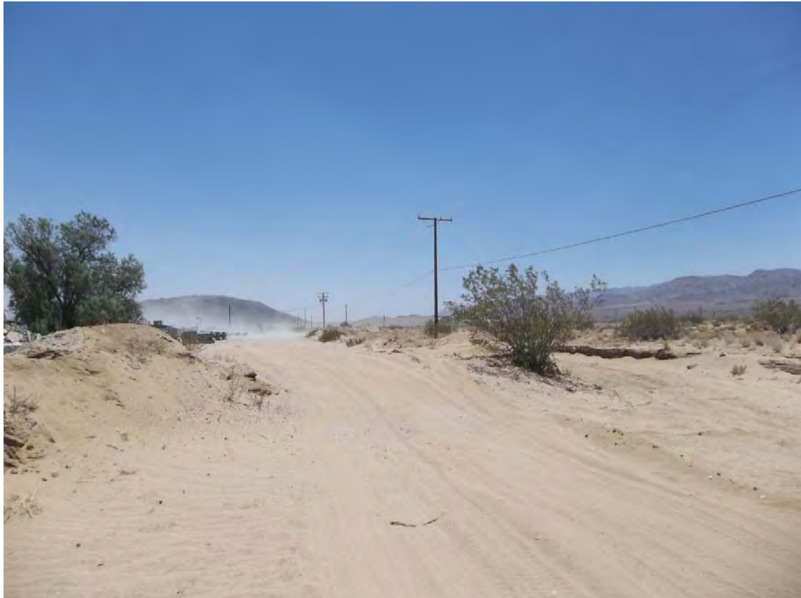
Photo 11: Offsite berm along south side of concrete plant (left side of photo) redirects flow away from the project site (channel to the right of the roadway).
