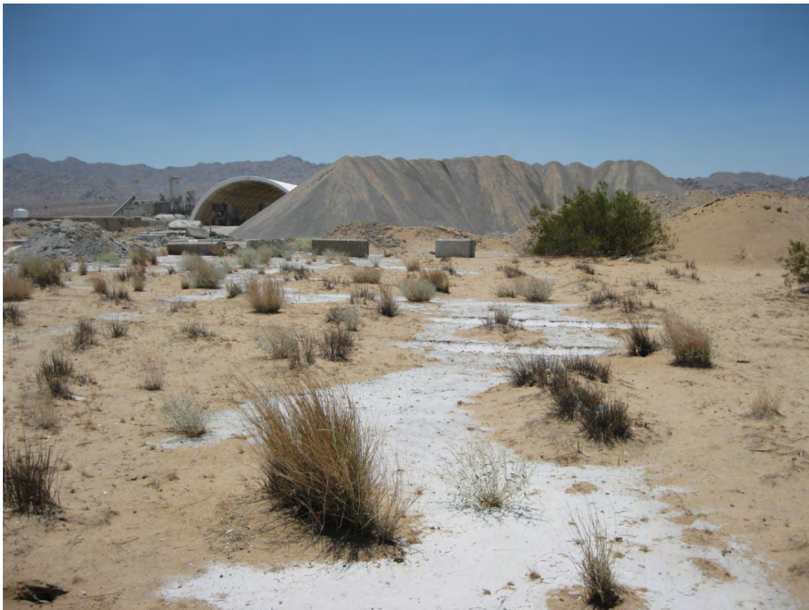
Photo 2: Runoff from concrete plant onto site, looking south.
