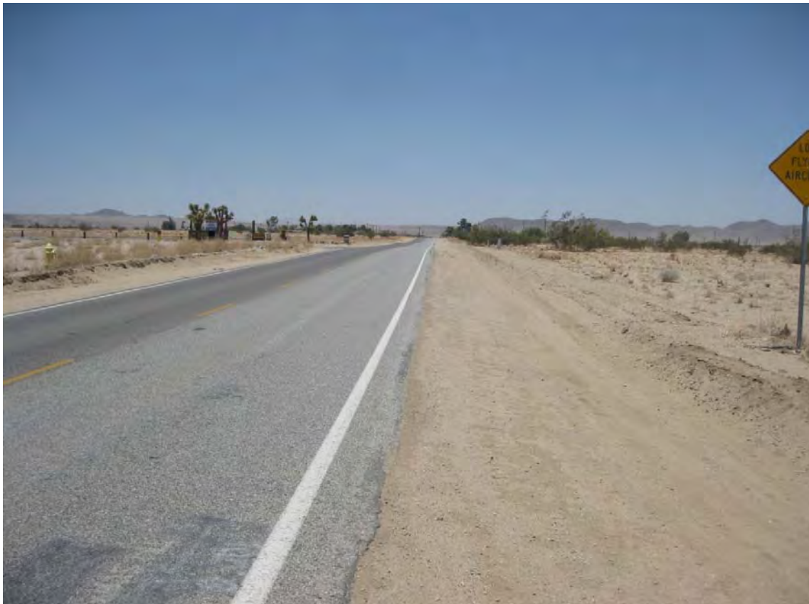
Photo 16: Graded shoulder along east side of Coyote Valley Road, directs stormwater flow to path pictured above, looking north.
