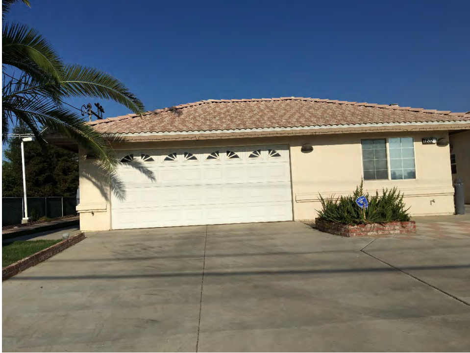
Photo 1 – View from Cactus Avenue looking towards the single-family residence at the southeastern corner of the Property (10532 Cactus Avenue).
