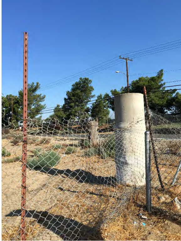
Photo 9 – Out-of-service flood irrigation concrete pipe on the northern edge of the Property.
