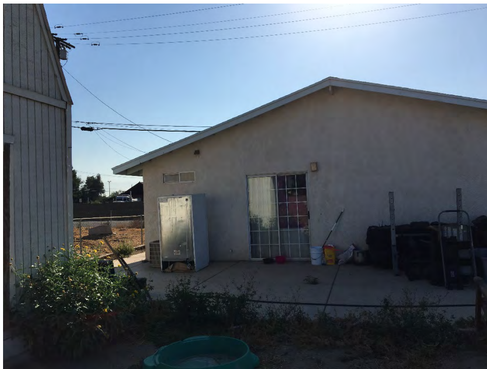
Photo 12 – The residence on the northeastern portion of the Property.
