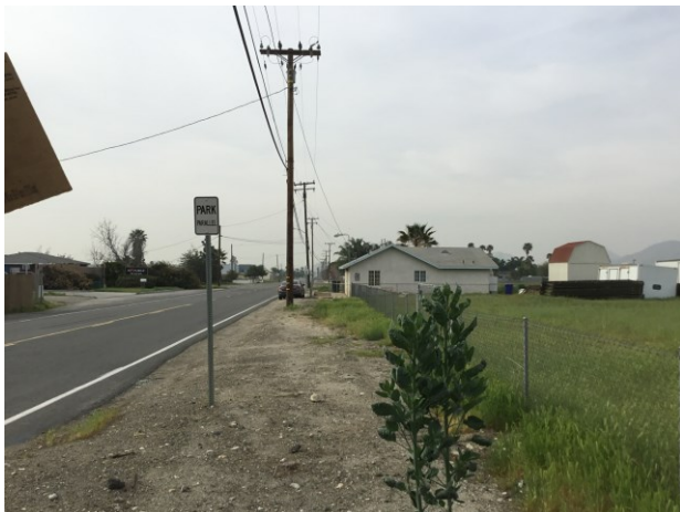
Photograph 2. Overview of the eastern project area boundary, including Cactus Avenue. Photograph taken from the northeast project corner. View to the south.
