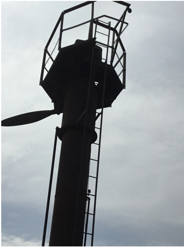
Photograph 12. Close-up of Windmill 1 from SCA-1.
