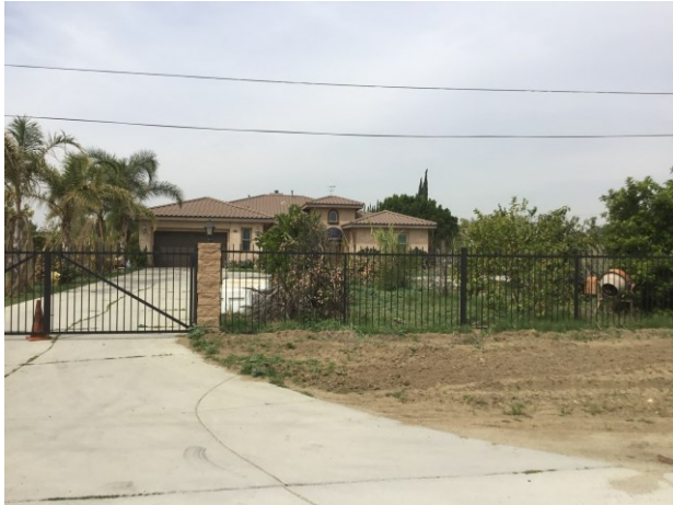
Photograph 5. West façade of the northernmost modern residence located along the western project area boundary. View to the east.
