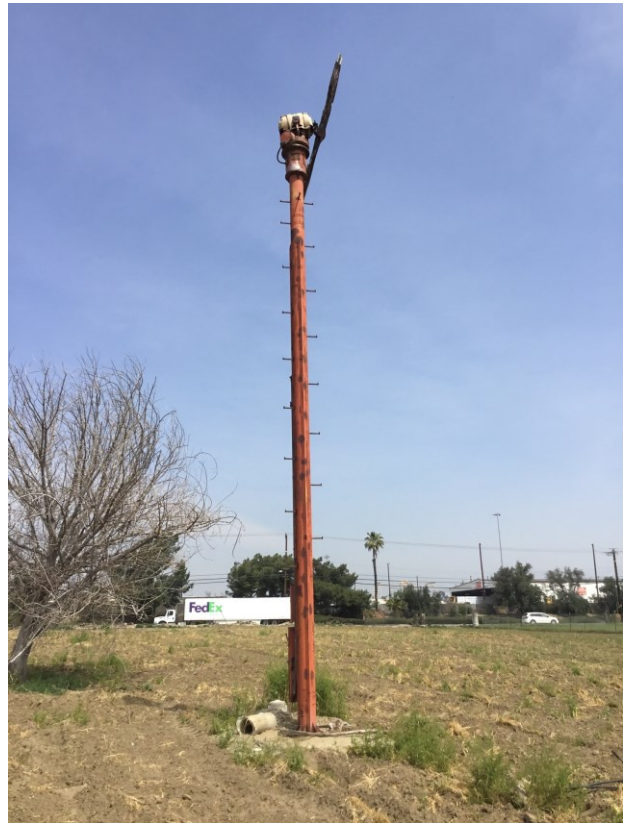
Photograph 13. Close-up of Windmill 2 from SCA-1.
