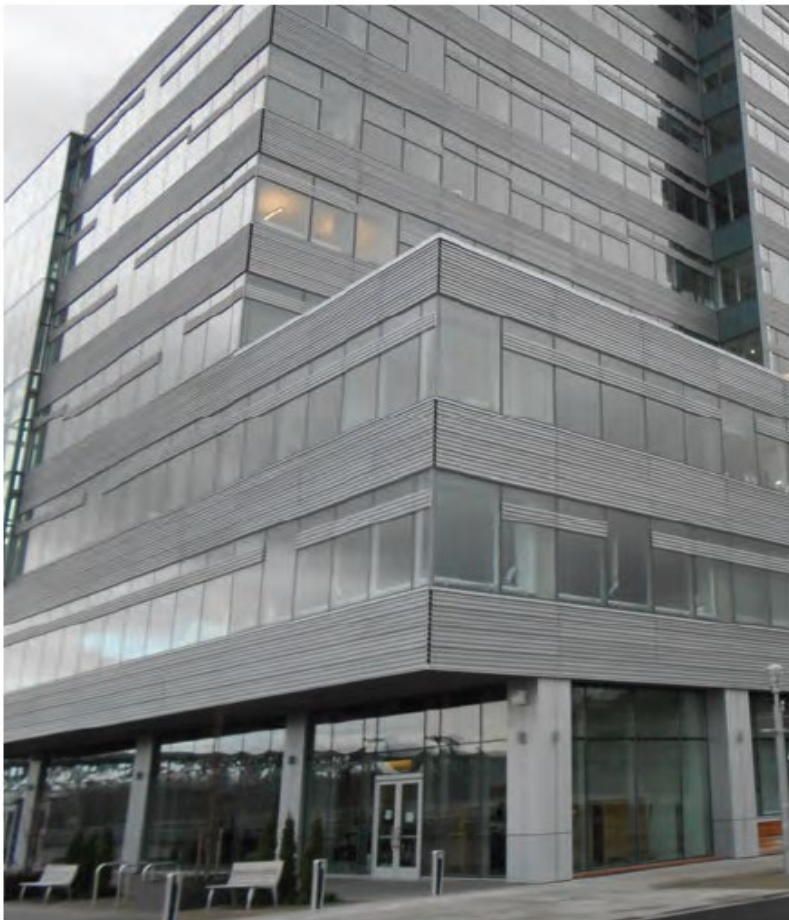
MCM use for cladding of an urban building.
