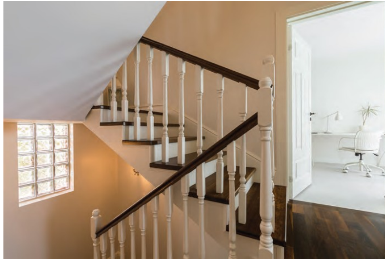
A passing handrail at a tread projection
