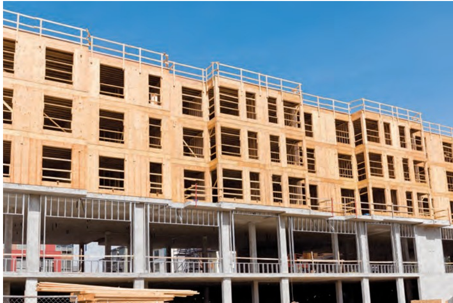
Building under construction
