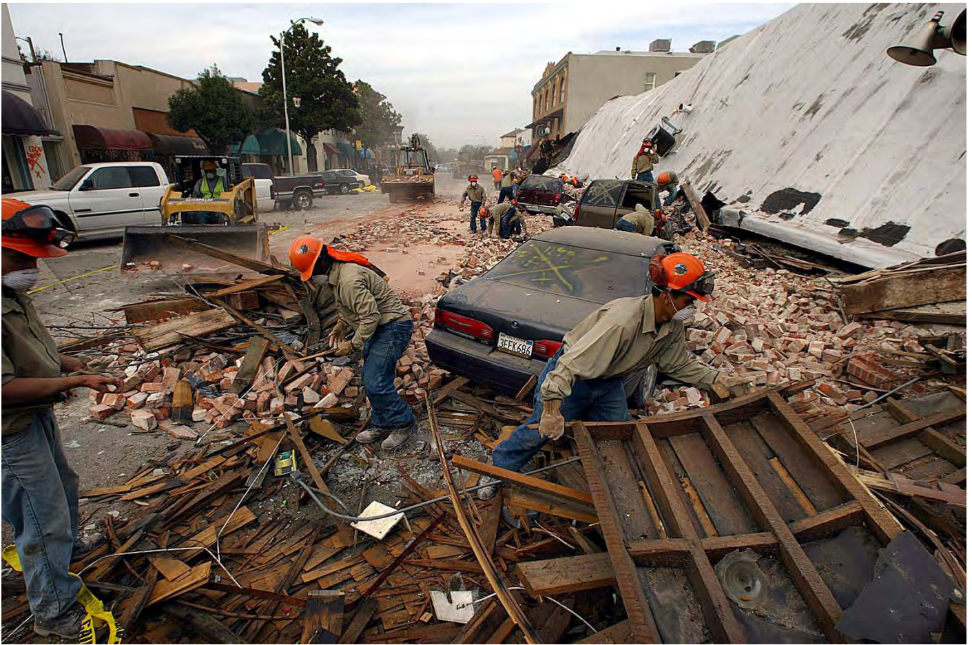
Rescue workers sift through the debris of an unretrofitted brick building in the wake of the 2003 Paso Robles earthquake. Two women who worked in the building died as they tried to flee. (Spencer Weiner/Los Angeles Times)
