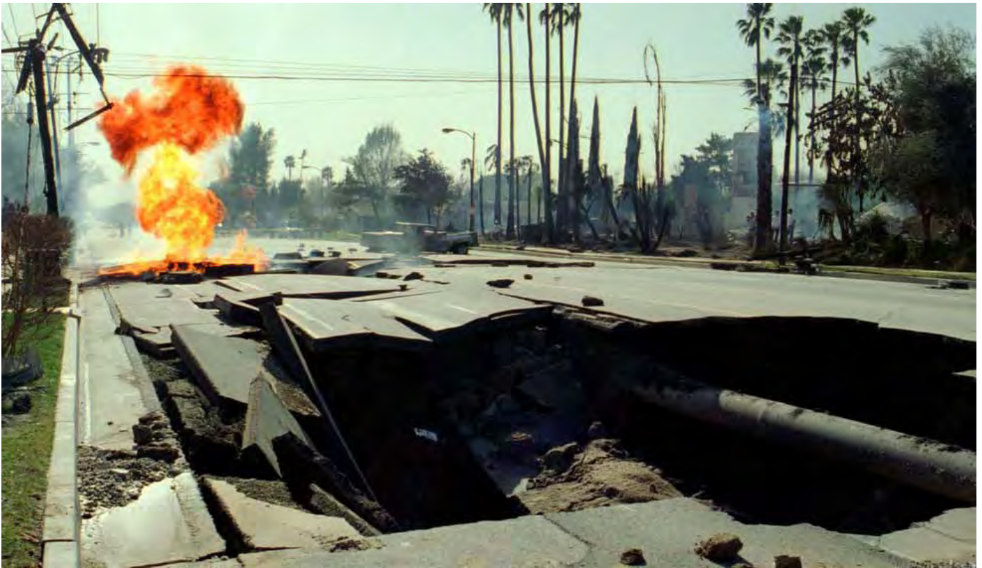
Flames billow from a ruptured gas main beyond a crater in the 11600 block of Balboa Boulevard in Granada Hills after the 1994 Northridge earthquake. (Patrick Downs / For The Times)
