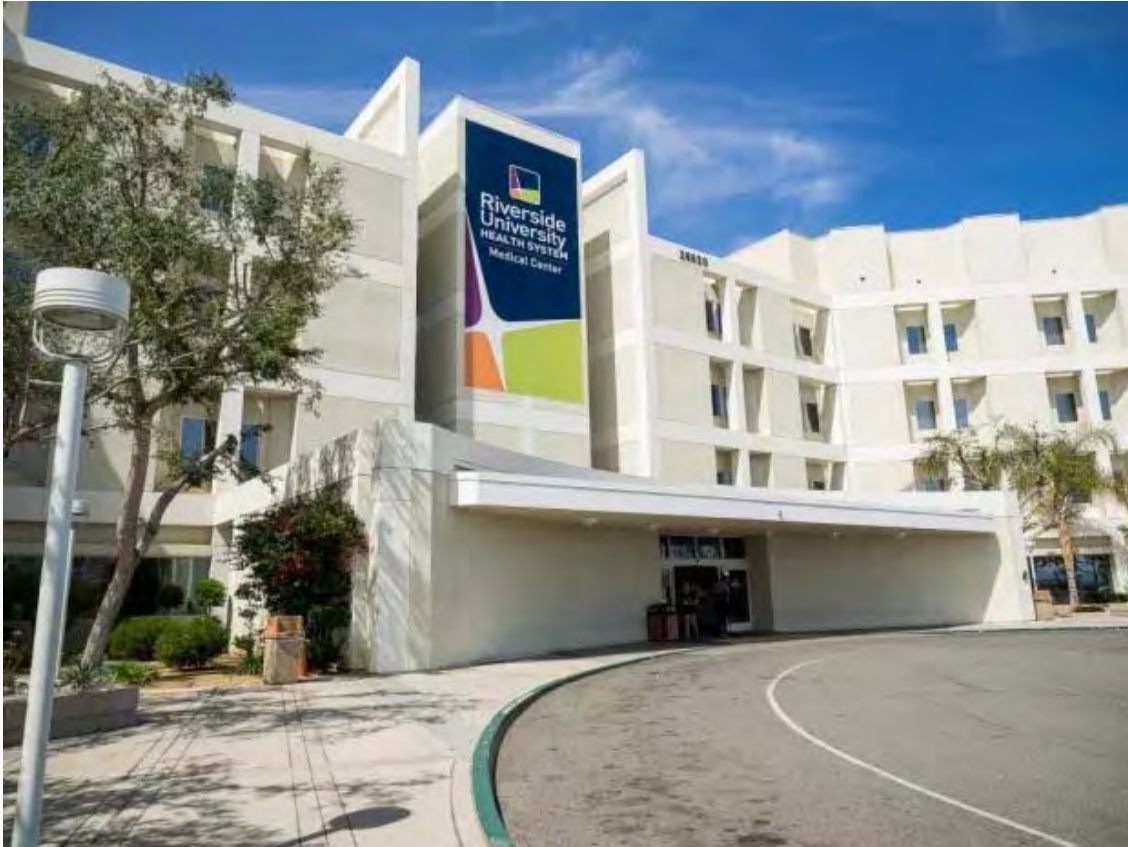
Riverside University Health System – Medical Center in Moreno Valley is just one of the services provided by Riverside County government.
