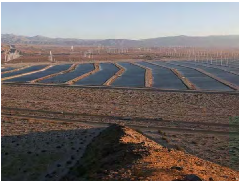
The ponds at the groundwater replenishment facility on the outskirts of Palm Springs are filled with Colorado River water. (Photo: Jay Calderon/The Desert Sun)
