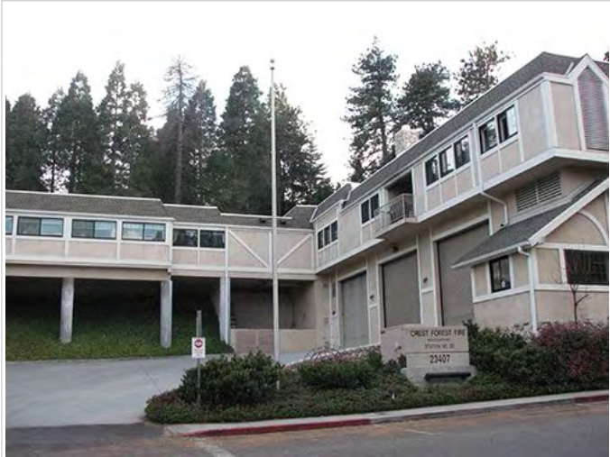
Crest Forest Fire Protection District headquarters building located at 23407 Crest Forest Drive, Crestline where the accident occurred (Photo by Gail Fry)
